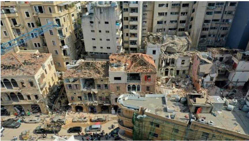
Fig. 18: Some examples of damaged buildings by explosion (AFP, 2020)
