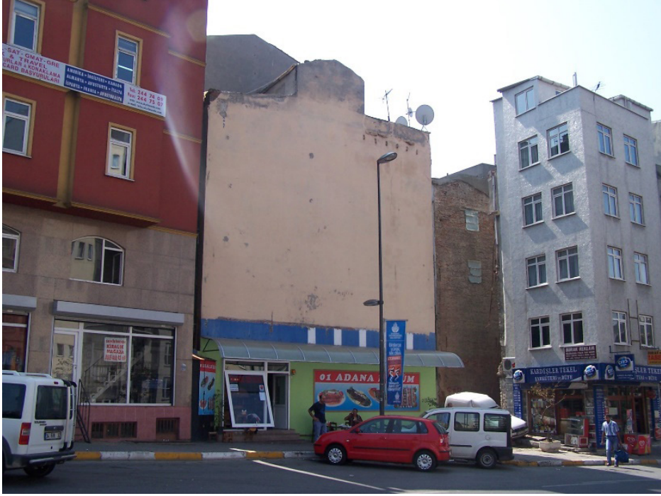
Fig.1 An example of bare wall façade in cityscape
