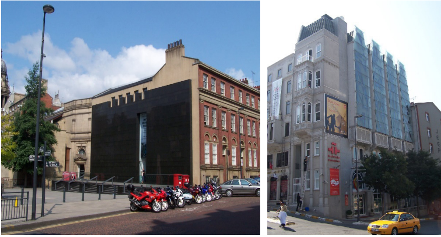
Fig.23 Examples of re-design in blank façades: (left) Henry Moore Institute, Leeds (UK), (right) Instituto Cervantes, Istanbul.
