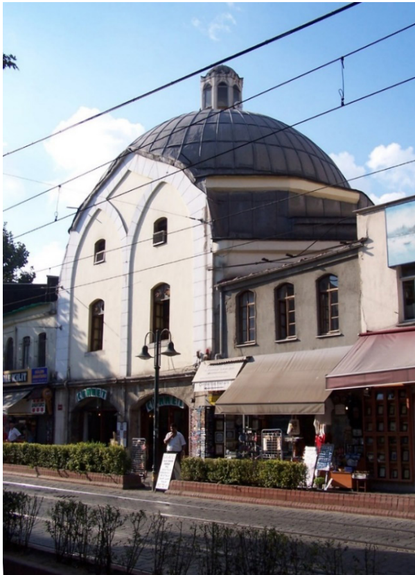
Fig.9 Re-designed façade of Cemberlitas Hamam in Divanyolu Avaneue
