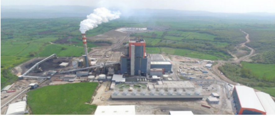
Figure 2: Çan 2 Local Coal Fired Thermal Power Plant.
