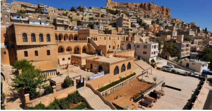
Figure 8: The silhouette of the city deteriorated by the addition of reinforced concrete structures. Source: http://www.mardinlife.com
