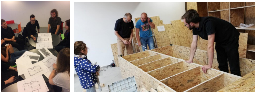
Figure 6. The stages of the work on the Po-Dzielnia project: a discussion with the Givebox activists about the concepts and the construction works carried out by the instructors, students, and voluntary workers. (photograph of K. Słuchocka)
